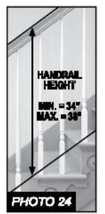
to walls. Students should inspect to be sure required handrails are actually available for users of the stair. Handrails are required on at least one side of the stair in homes and on both sides in schools and public buildings. Handrails should begin at or before the start of the stair and extend to or beyond the top step.
