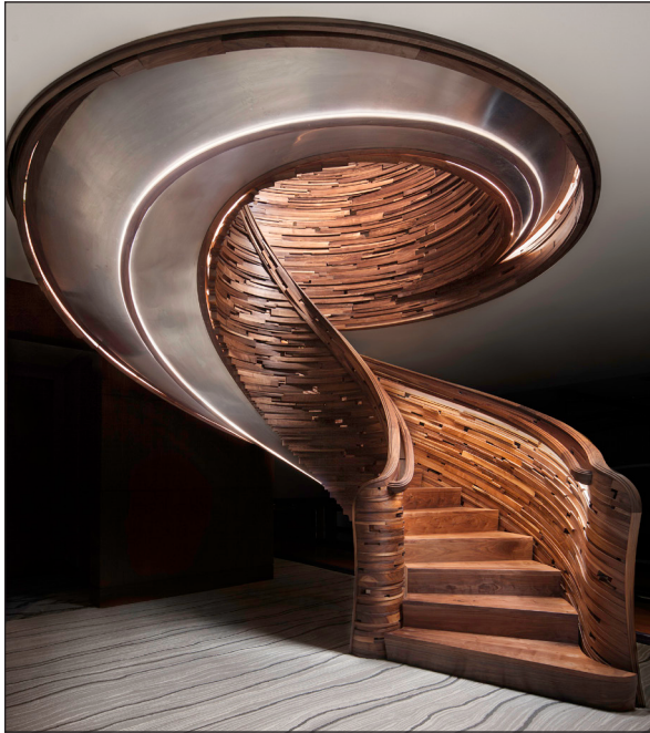
Laminated hardwood curved staircase that incorporates a large variety of species for architectural effect.
